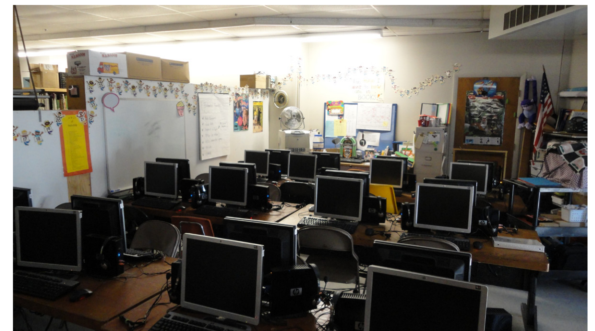
Lack of space in the Media Center and the Computer Lab is compounded by poor acoustic separation to render these areas inadequate for educational needs. Reconfiguration and renovation could remedy these issues.
