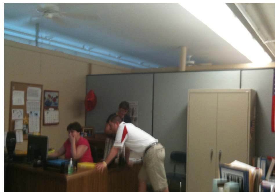
Partial height walls dividing the main office from student intervention areas provide for no acoustic separation. Similar conditions existing in many areas of the school.
