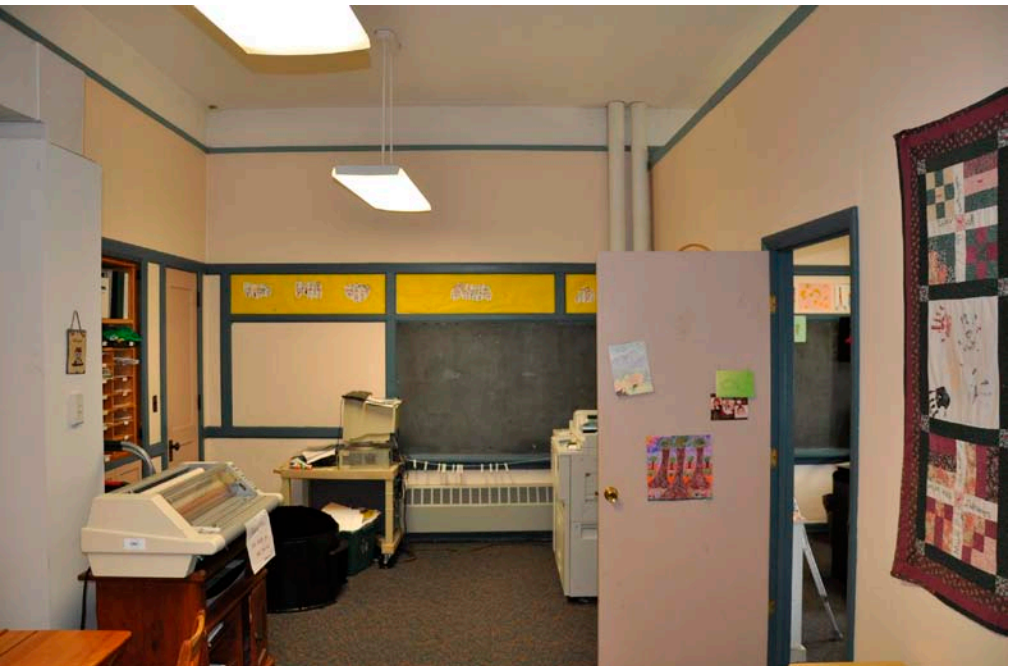
The Main Office area, including the Principal's Office do not achieve acoustic separation as the partitions do not extend all the way up, offering no privacy.
