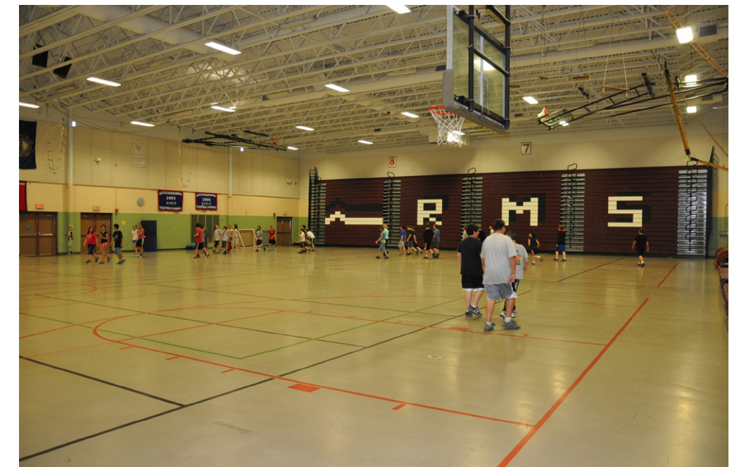
Some areas, like the gymnasium, lack natural light. To remedy this, diffuse lensed skylights could be provided, along with daylight harvesting sensors, to both improve lighting and provide energy savings. Cost effective solutions include packaged round skylight units (such as Solar-tubes), small rectangular packaged units, or pyramidal skylight units.
